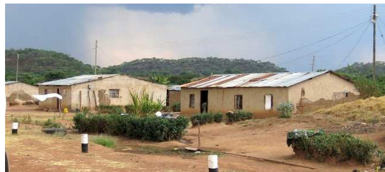
ZNS Kalenda Farms, Electrified Staff Houses
