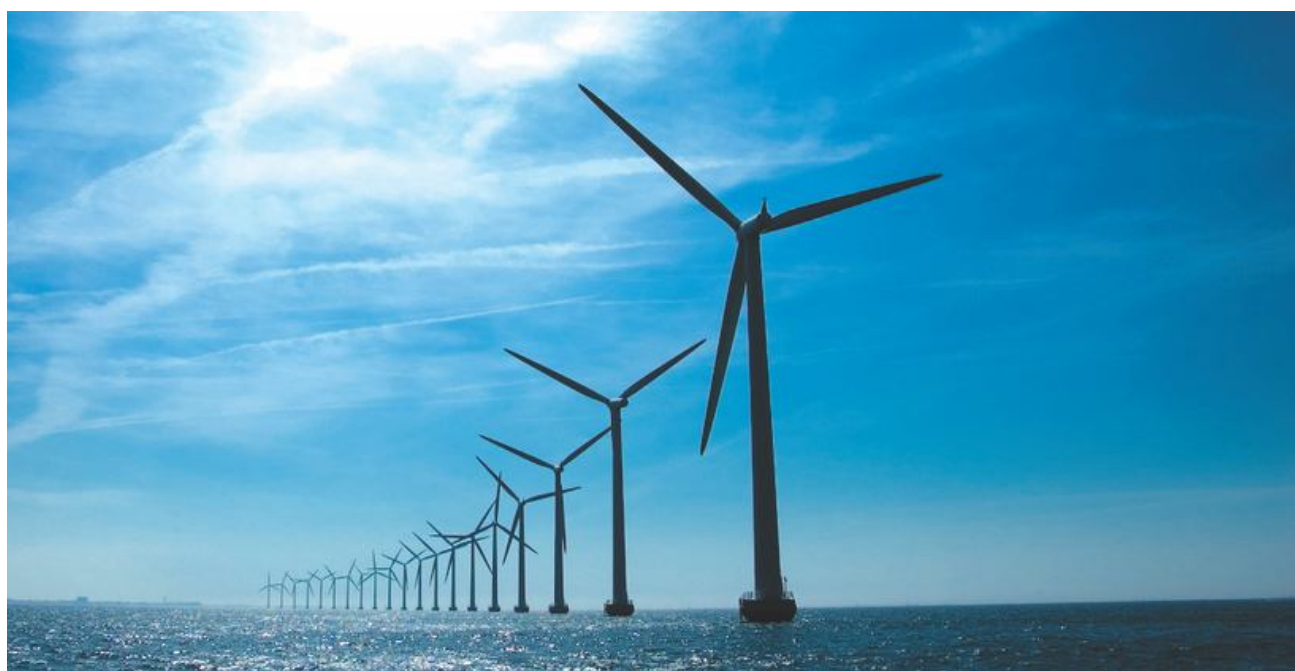
Offshore wind energy has potential in India
