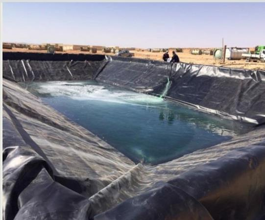
24 contaminated tanks were treated and the wastewater pumped into an evaporation lagoon.
