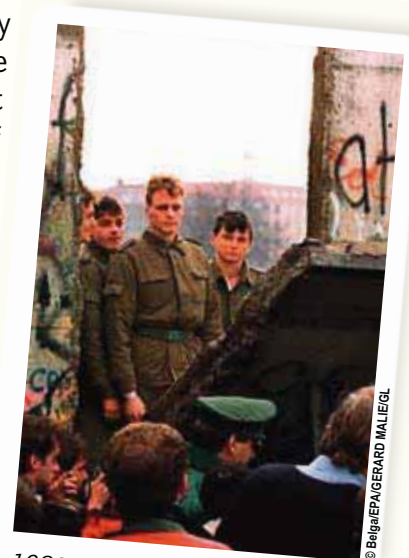
1989: demolishing the Berlin Wall.
