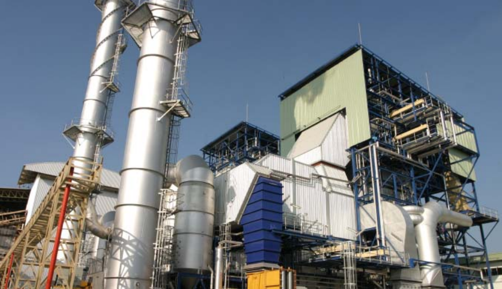
An EU-funded power plant in northeast Thailand turns sugarcane residue into electricity.
