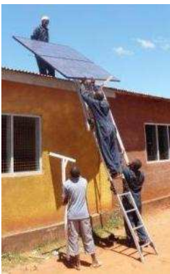
Setting up of a solar system
