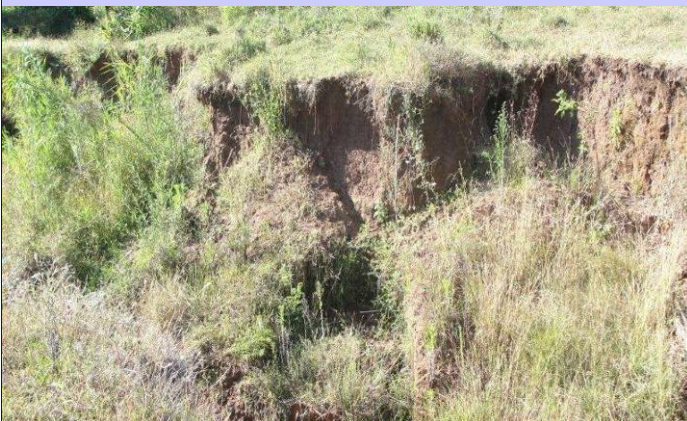
An area affected by erosion at Mwansekwa area in Mbeya
