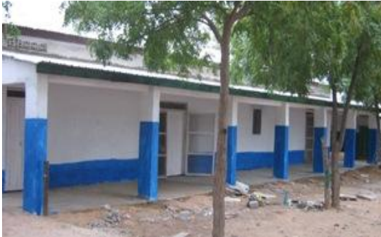
Building with Operation Theatre after rehabilitation
