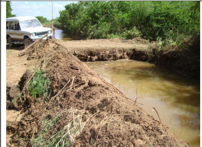
Rehabilitation of one side of Buffow Canal
