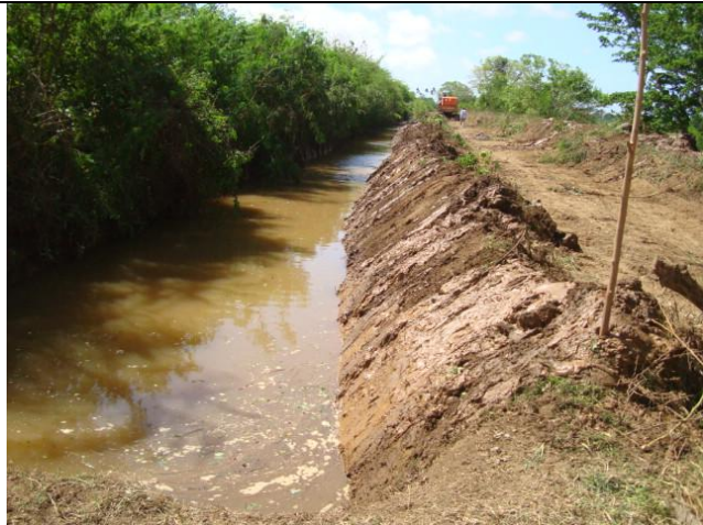
Rehabilitation of one side of Buffow Canal
