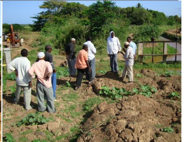
Buffow canal off-take from Cesare Maria Canal (before rehabilitation)
