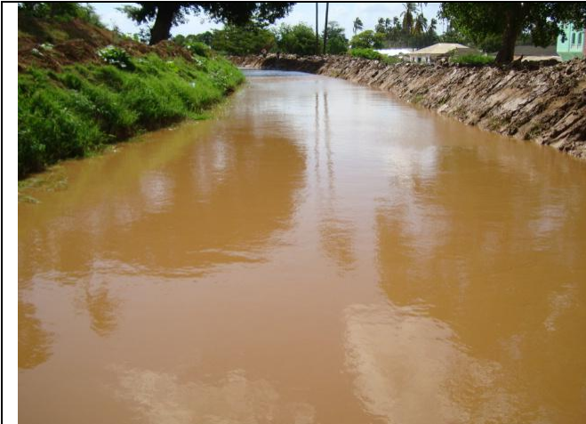
Rehabilitation of one side of first section of Cesare Maria Canal
