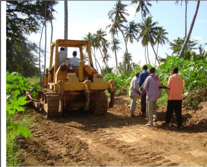
Cutting of embankment before canal excavation
