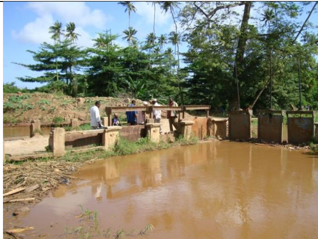
Off-take of Cesare Maria Canal from River Shabelle (before rehabilitation)
