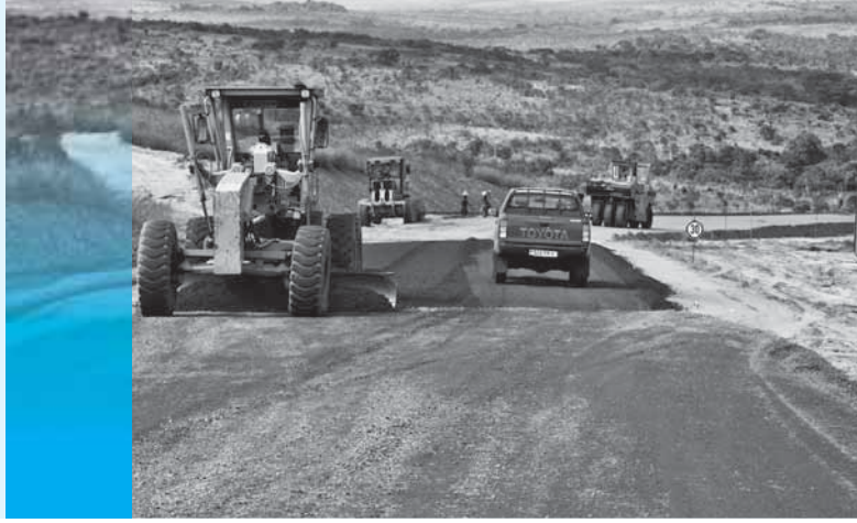
Construction d'une route Congo © CE/Claudio Bacigalupi
