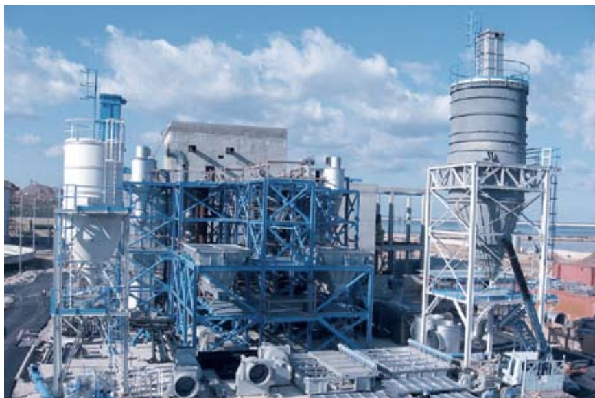
"Kesrwan Water and Wastewater" project, funded by the EIB loan together with NIF technical assistance.
