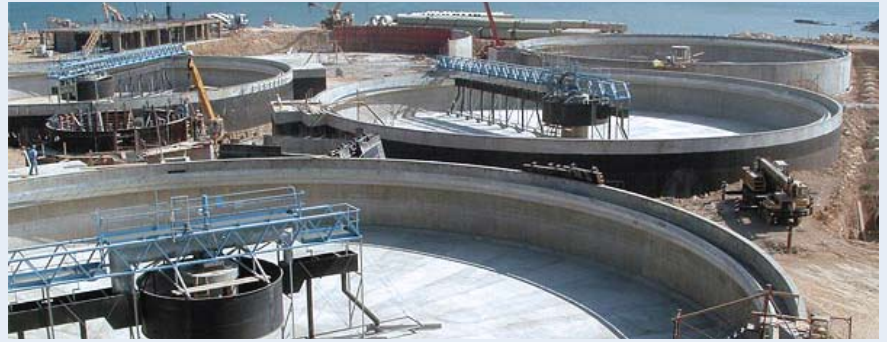
Tripoli wastewater treatment plant (financed by the European Investment Bank).
