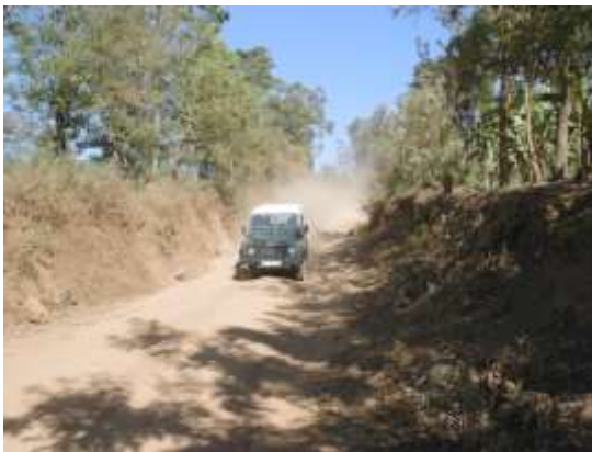
Before and after: the Meru to Marimba road that was completed in December 2013.
