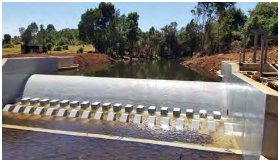
Weir for water intake on Chamara River
