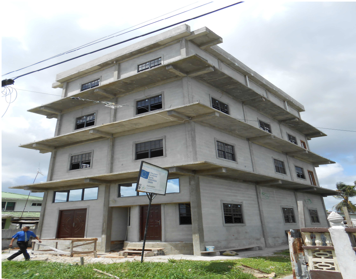
Multi-purpose building under construction
