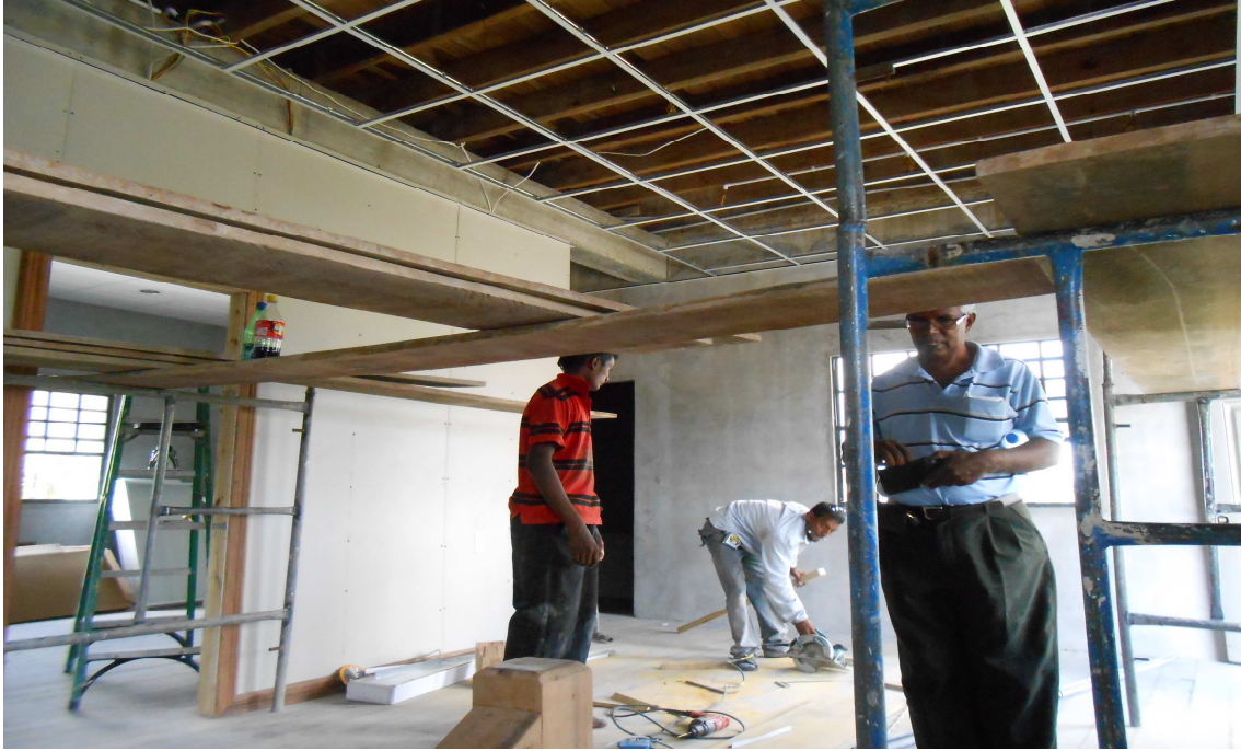
Works under way inside the multi-purpose building
