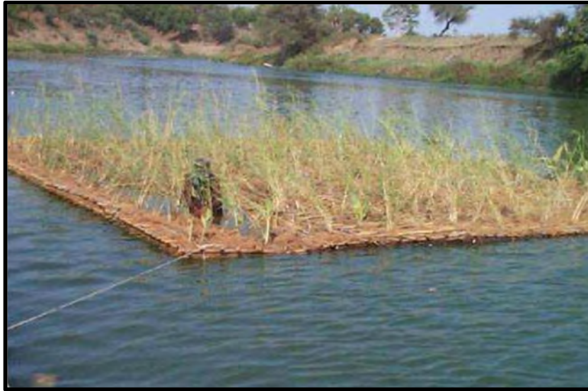
Figure (39): Floating wetland installed on the river Kshipra-India
