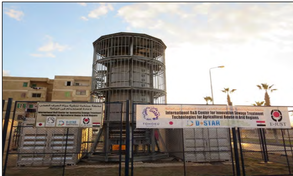
Figure (11): Pilot Scale plant in Borg Al Arab city-Alexandria
