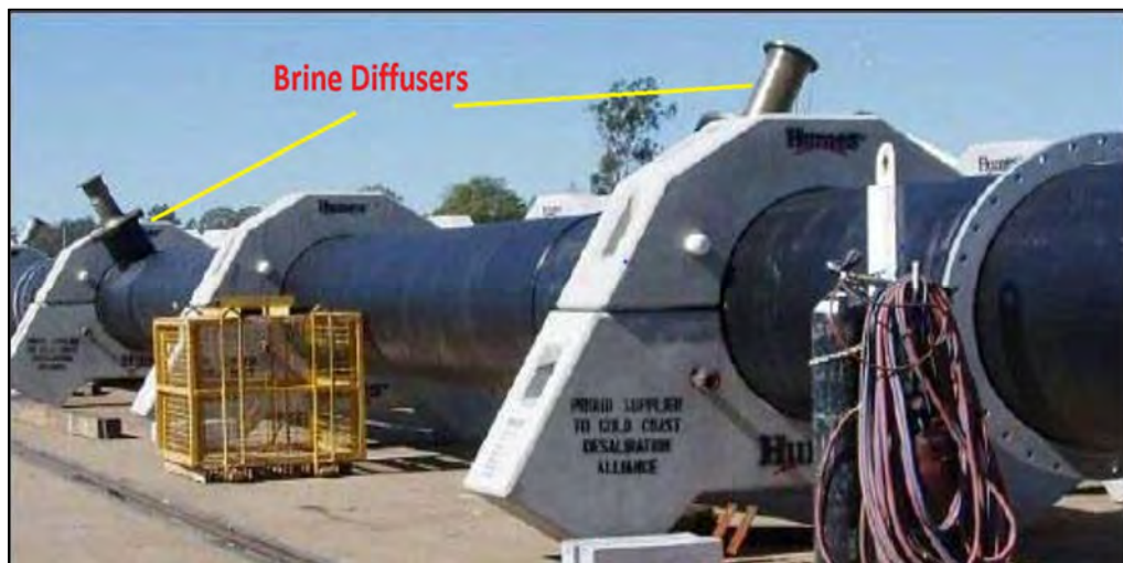
Figure (8): Brine diffusers
