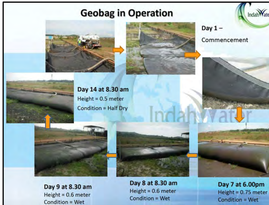
Figure (41): Geobag usage in sludge dewatering
