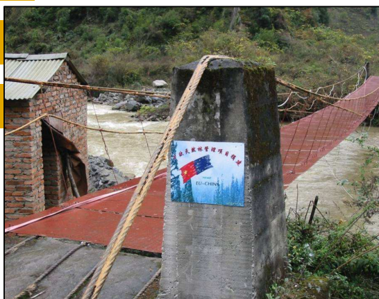
Fig. 5 A suspension bridge rehabilitated in Pingwu
