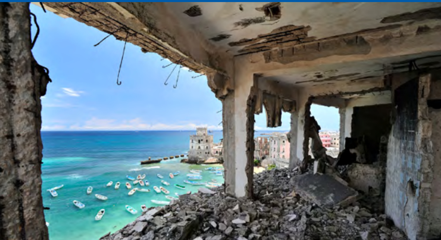
Once one of Mogadishu's most luxurious hotels, the Al-Uruba lays in ruins after two decades of civil war. Though building work in Mogadishu is on the rise, it may still be several years before many of the city's buildings will be restored. AU-UN IST PHOTO / TOBIN JONES.
